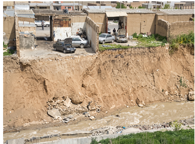
Fig. (2). Construction on the river route.
