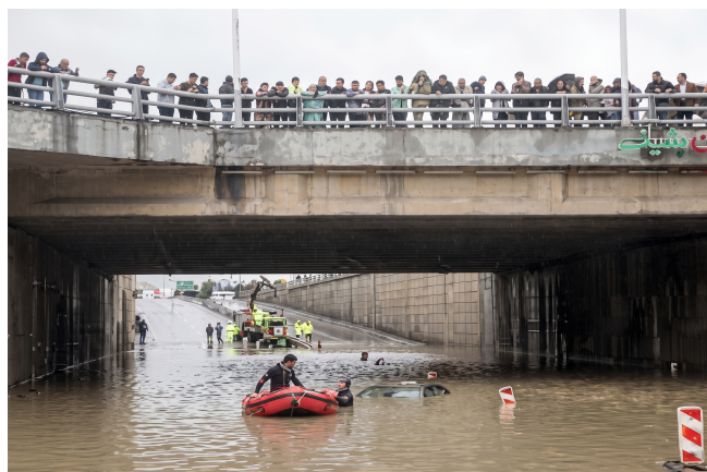
Fig. (16). People gathering at the site of the incident, increasing the risk of collapse of the overpass bridge due to heavy rainfall.
