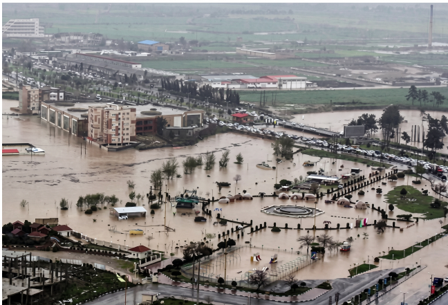
Fig. (19). Inadequate urban structure in directing surface water.
