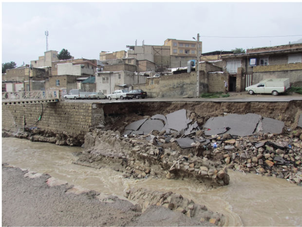
Fig. (8). Demolition of the retaining wall and the river by-pass.
