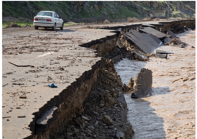
Fig. (10). Construction of roads on the riverbank.
