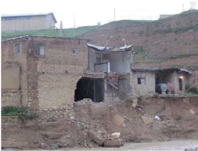
**Fig. (7).** Foundation scouring and collapse of the load-bearing walls and roof.
