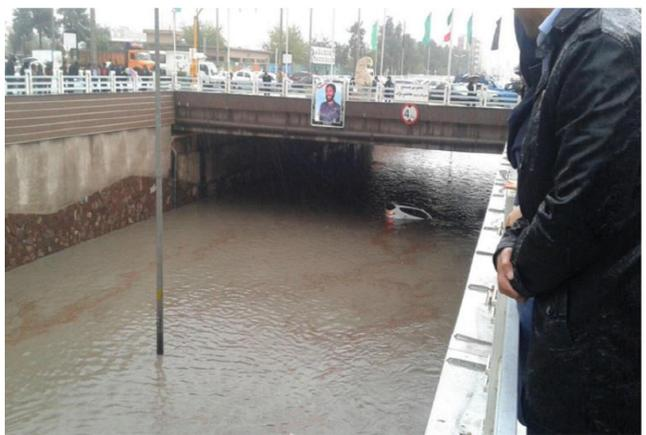
**Fig. (11).** Construction of an underpass without considering the drainage system of the water entering the underpass, the steep slope of the underpass, and the accumulation of inlet water.
