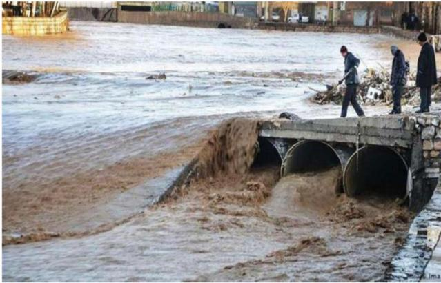
**Fig. (12).** A narrow path being created for the waterway due to the construction of a bridge and its narrow span.
