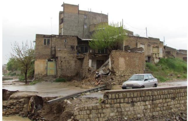
**Fig. (4).** Residential buildings lacking design considerations for flood load and proper technical specifications are more vulnerable along the flood route.
