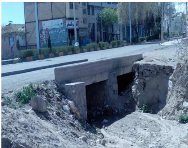
**Fig. (14).** Bridge openings are blocked.
