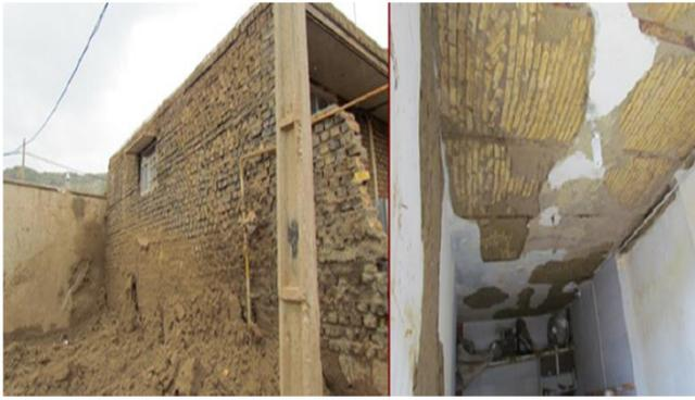
**Fig. (6).** The building with a load-bearing wall system supported by a steel coil and a rough brick arch roof; the adjacent building, which lacked a suitable structural system, was destroyed.
