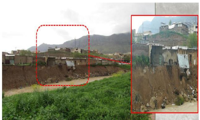
**Fig. (5).** Residential construction along the river upstream route, which has scoured the foundation and destroyed the buildings during the flood.
