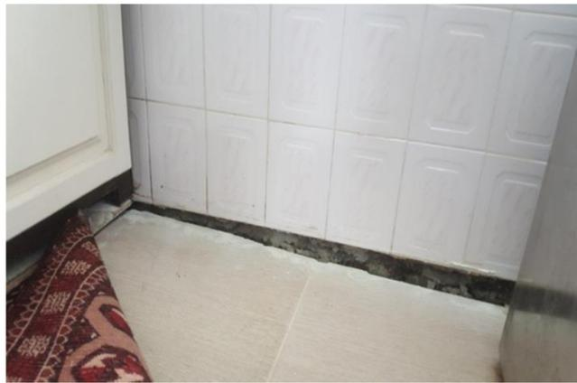
**Fig. (13).** Excessive settlement of the kitchen floor due to the use of soil instead of rubble (blockage).
