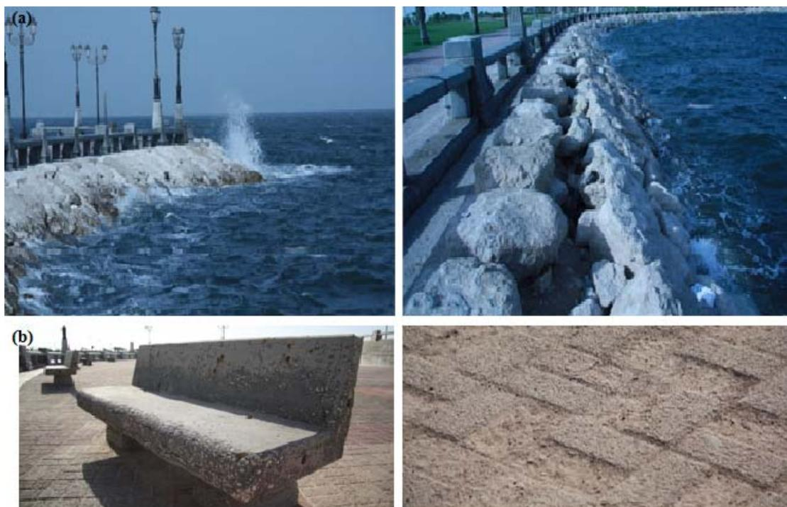
**Fig. (4).** (a) This segment is subjected to strong waves due to disappearance of intertidal zone (b) Effects of huge swash on the site furniture and paved surfaces along this segment.
